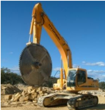
C. Single disk saw on an excavator
